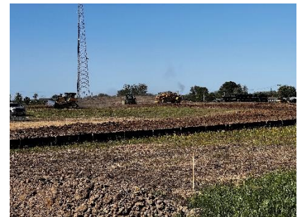
Site Work, Humble Robinson Spec. Building.
